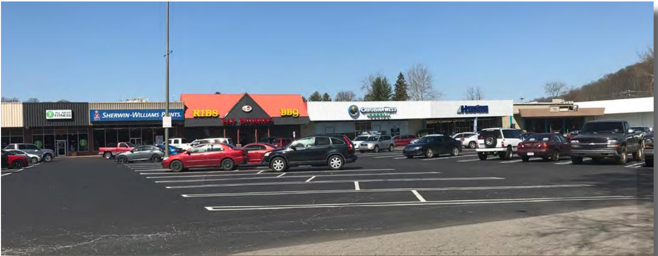
Above: The large impervious surface provides opportunities for infill development at Waynesville Plaza main shopping center to create additional commercial and residential spaces. Infill could create a Main Street feel similar to Waynesville's historic downtown.
